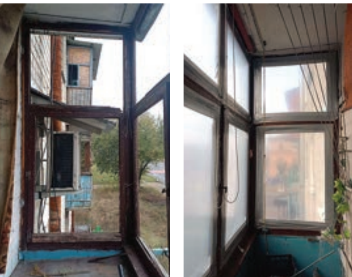
Before and After: Left, shattered windows in a Ukrainian home in Izyum, a city in the Kharkiv Oblast. Right, the same home with new insulating windows. (Photos courtesy Insulate Ukraine )
